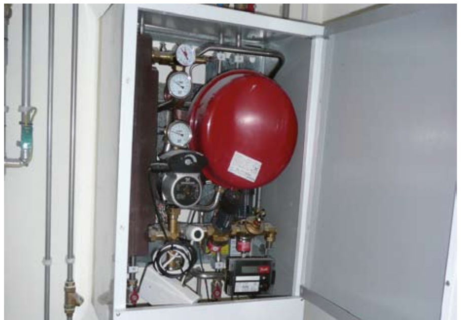
.Danfoss Termix VVX flat station.
