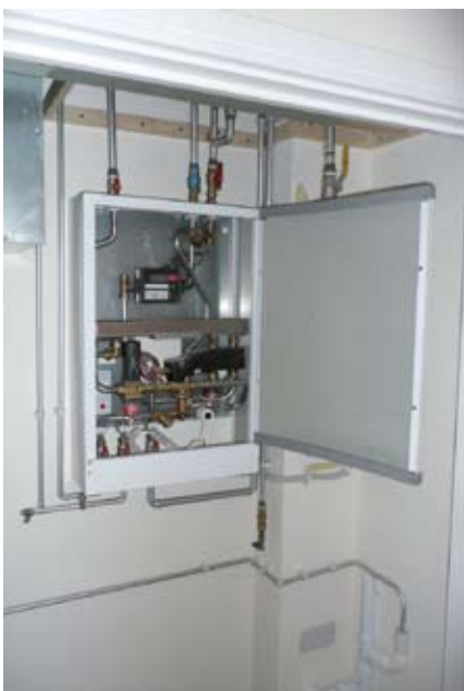
Danfoss Termix VMTD-F flat station.
